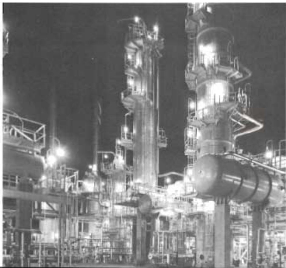
Naphtha fractionation unit at the Altona petrochemical complex. Mobil Oil Australia Ltd
